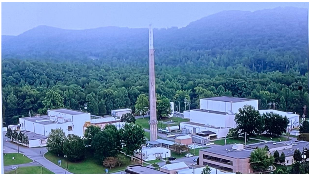
Aerial photograph of the High Flux Isotope Reactor and the Radiochemical Engineering and Development Center, where transuranium elements produced at HFIR are chemically separated and prepared for shipment.
